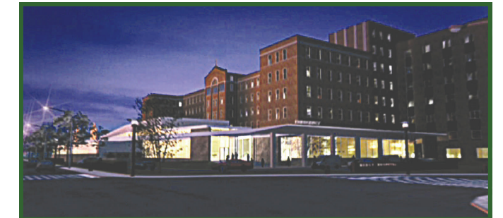
The new face of Mercy Hospital.
